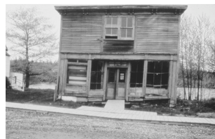
The store, before work began.
