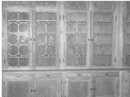
Built-in bookcases are fronted with mullioned glass doors in the second floor suite, formerly occupied by Roman Catholic Archbishops of Halifax.
