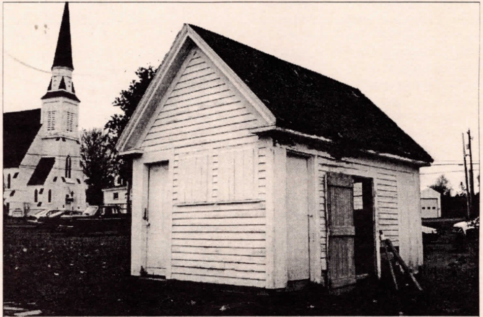
Great Village School outhouse, before the move. The centre door on the right was added while it did shed duty.
