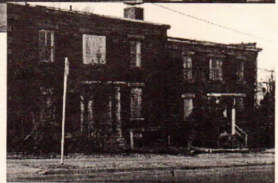
Top: Mid-May, 2000 and progress is evident
