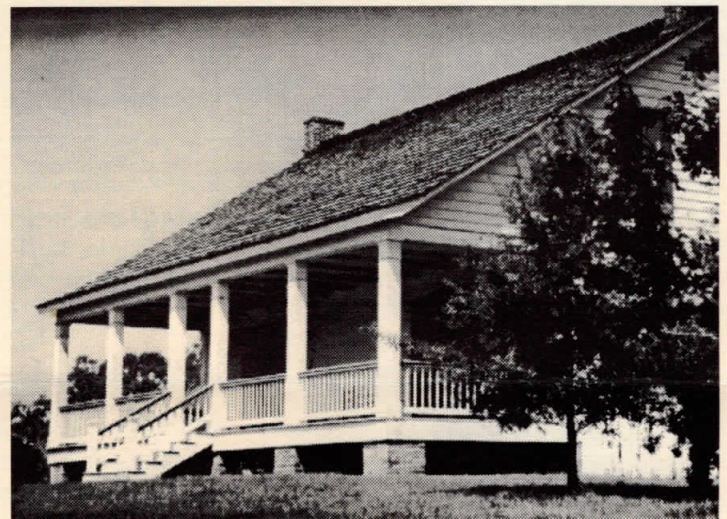
A classic "Cajun" cottage. This style appeared among the Acadian or "Cajun" population of Louisiana in the early 1800s and became a prototype. Most Cajun homes followed this pattern until the 1930s.
