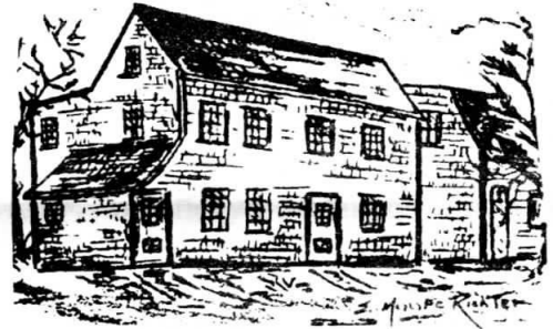
Historic Quaker House
